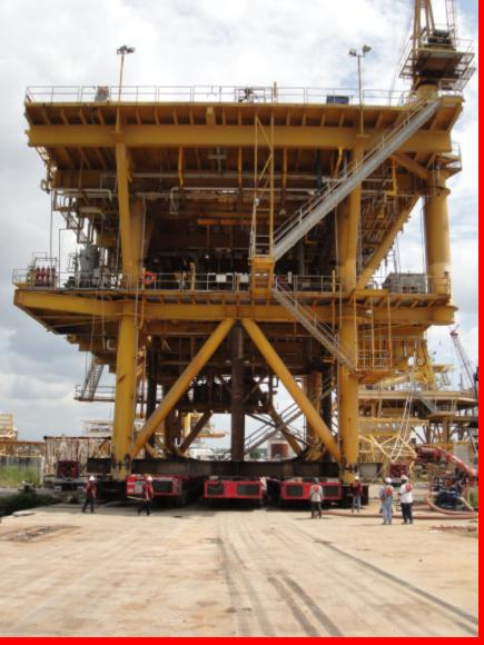
Measuring 160' x 80' and weighing 1650 tons, the Berard Team used sixty lines of spmts consisting of a mix of both SLE's and ESE's. The massive deck was offloaded from a 260 x 72 deck barge into customers yard. Once in the yard the deck traversed over inadequate ground conditions and involved several tight turns. Once again the manuverability of the spmt's came through to make this collossal project another success story for Berard.
